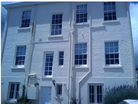
Back of building
